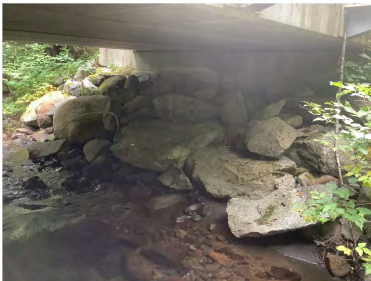
Right Bank Abutment when facing downstream
