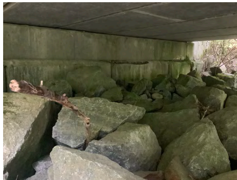
Left Bank Abutment when facing downstream
